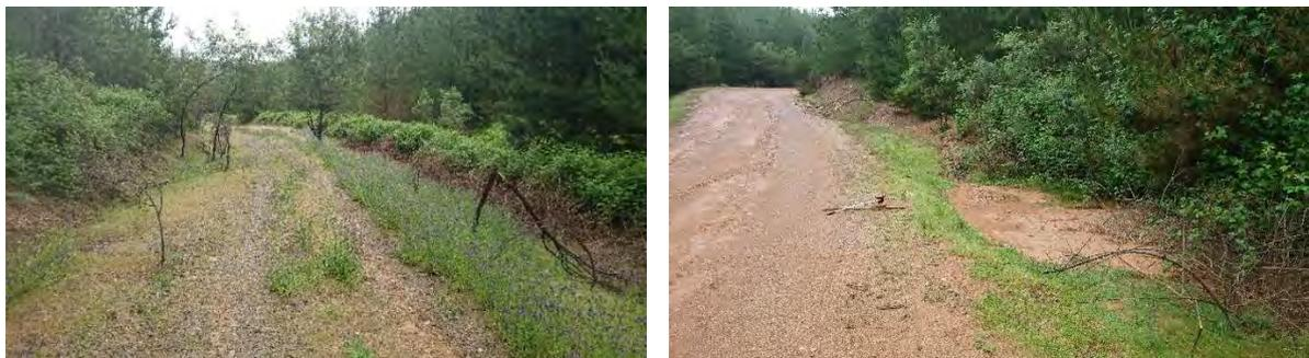
**Figure 10.** Left- Example portion of partially overgrown portion of road in Carabost State Forest, right- Example table drain dispersing flow and depositing sediment in a flat area adjacent hillslope the road has been cut into.
