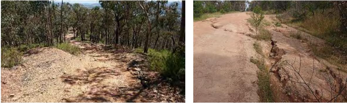
**Figure 4.** Top- Example of cross- bank and mitre drains on ridge crest in the Wereboldera State Conservation Area, bottom- deeply rutted road surface that causes flow to bypass an upslope drain.
