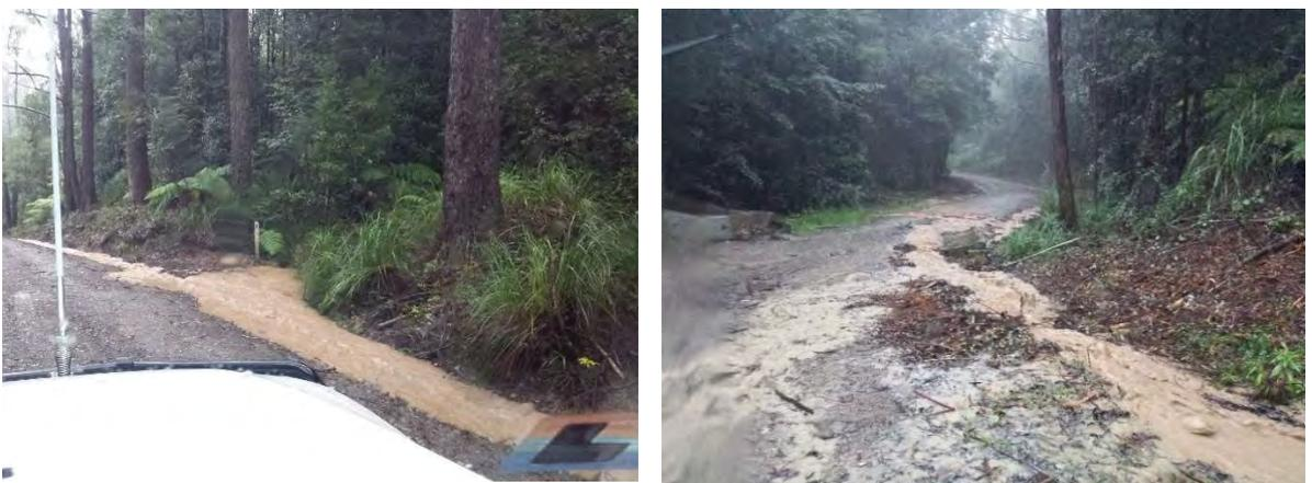
**Figure 32.** Examples of road-related erosion. (left: Photo Ross Peacock) Road runoff overwhelms culverts (left) and transports sediment and debris downslope (right: Photo Ross Peacock)
