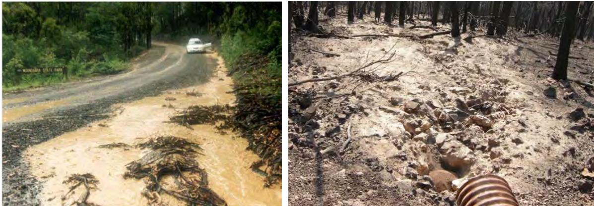
**Figure 31.** Examples of road-related erosion. (left: Photo Gary Sheridan) Road runoff and detachment of sediment from the road surface. (right) Hillslope erosion caused by discharge from the road surface after a bushfire.
