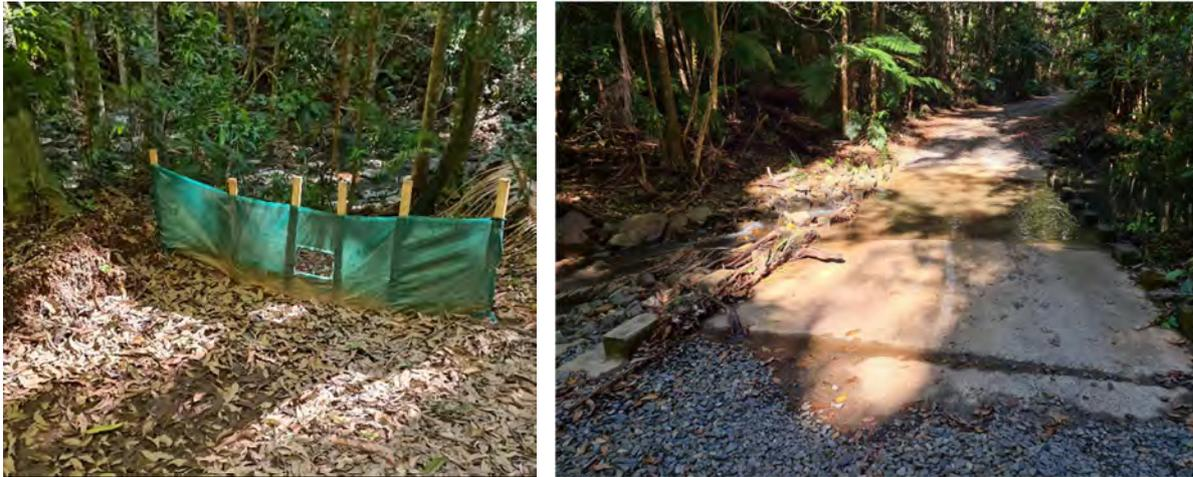
**Figure 18.** Left – example of a silt fence installed to intercept flow from a drain that directly connects with a waterway, Yarriabini National Park, right- example crossing.
