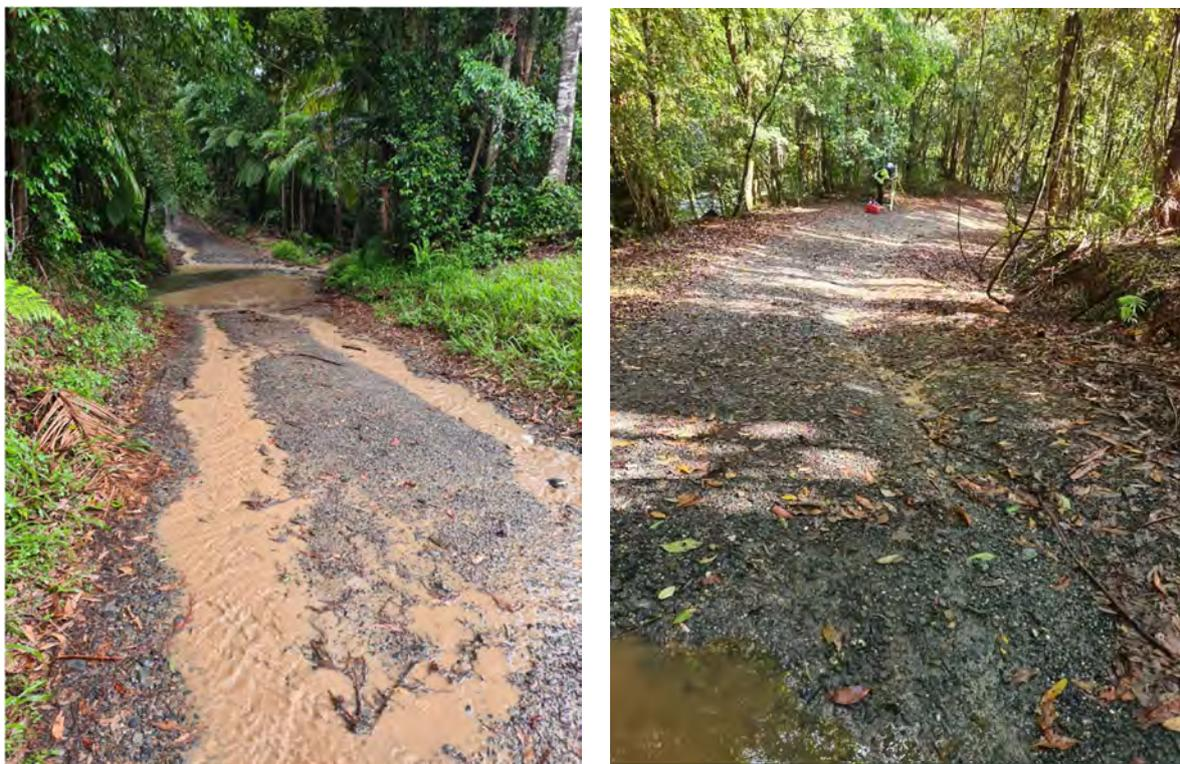
**Figure 16.** Left- Example of sediment-laden runoff flowing into a ford type waterway crossing in Bindarri National Park, right- steep section of road upslope from the waterway crossing at left.
