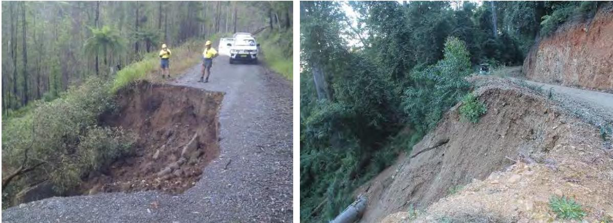
**Figure 33.** (left) Example of a road constructed in the 1950s using side-casting techniques (where excavated material is simply pushed over the edge of the roadway), and has collapsed during large precipitation event in 2013 (Photo FCNSW). (right) Failure in road batter located in a very steep hillslope in response to east coast low heavy precipitation event (441 mm in 3 days)
