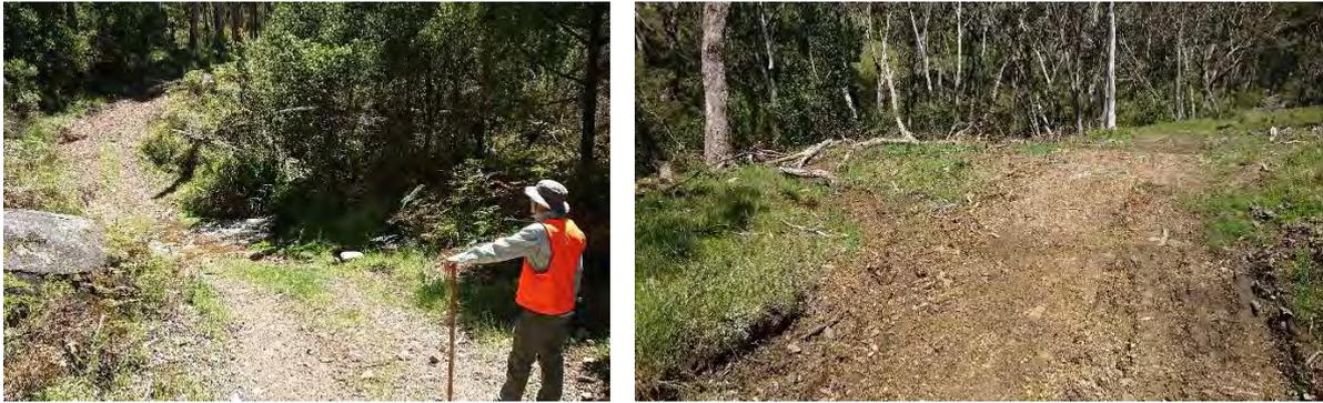
**Figure 6.** *Left- A steep approach to a waterway crossing (ford) along Buckleys Trail, and right – example of a mitre drain dispersing flow down slope.*
