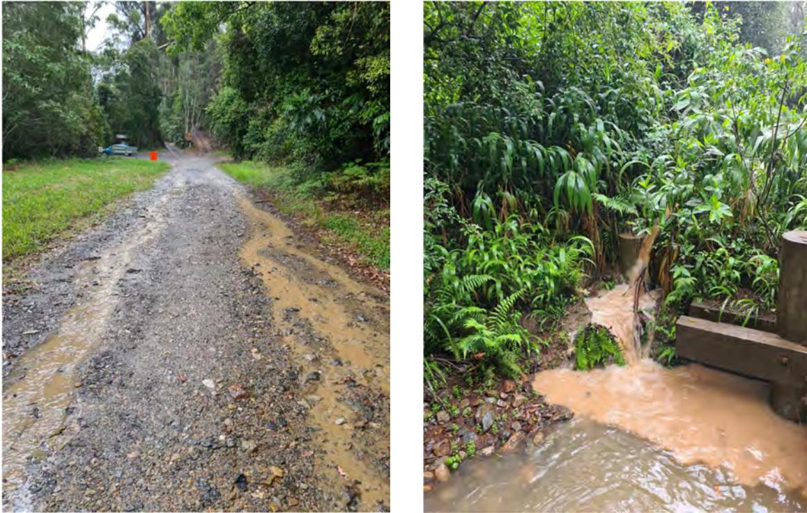
**Figure 14.** *Left -Example segments of road surveyed in the Orara West State Forest and, right – A drain directly connected to a waterway at a crossing, discharging sediment laden runoff a waterway in Orara West State Forest.*
